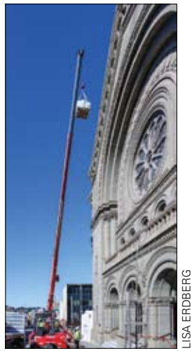
A crane hoists roofing material to the dome.
