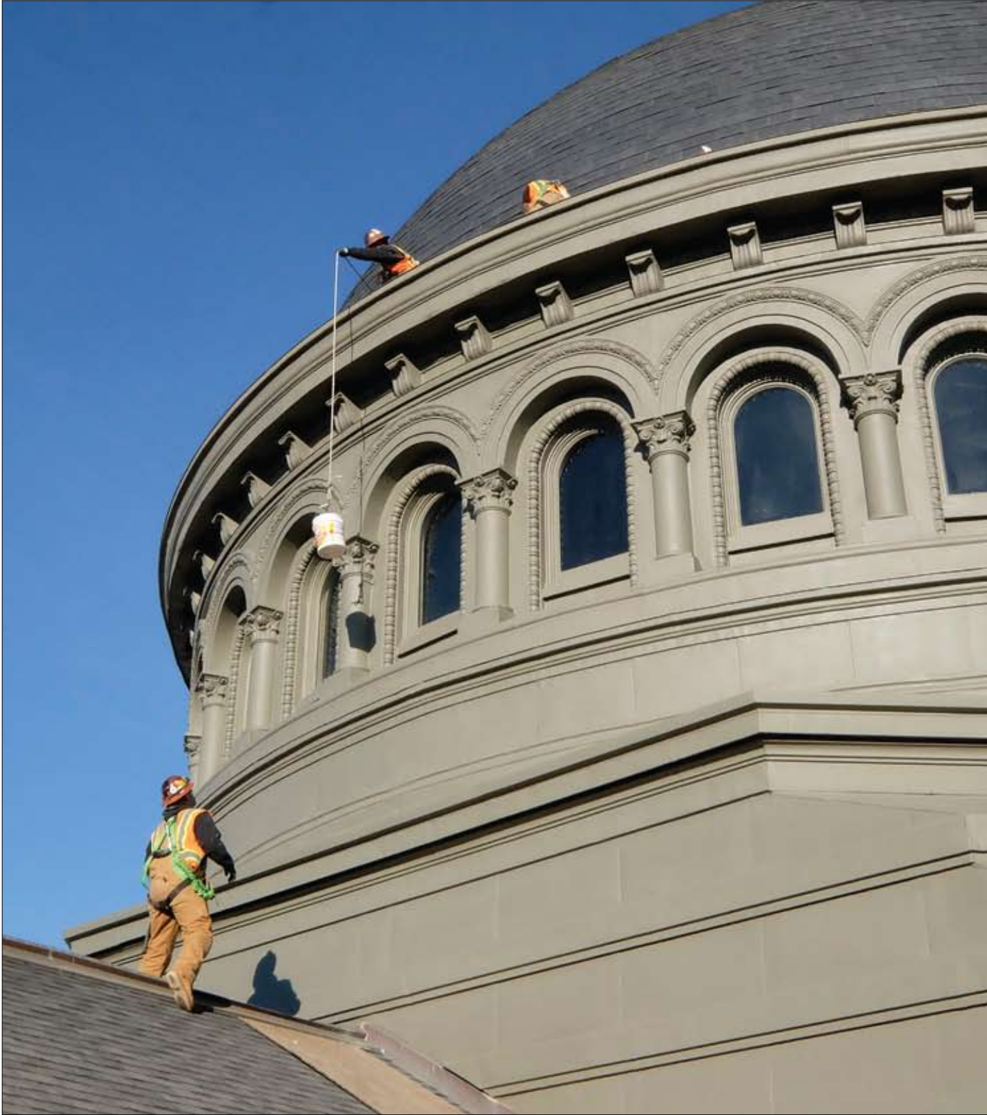
Workers lift a bucket of rivets up to Sherith Israel's dome (above) as part of the seismic retrofit project. Inside, workers reinstall one of the building's stained glass windows (below left) and get a lesson in the sanctuary about the building's rich history (below right).
